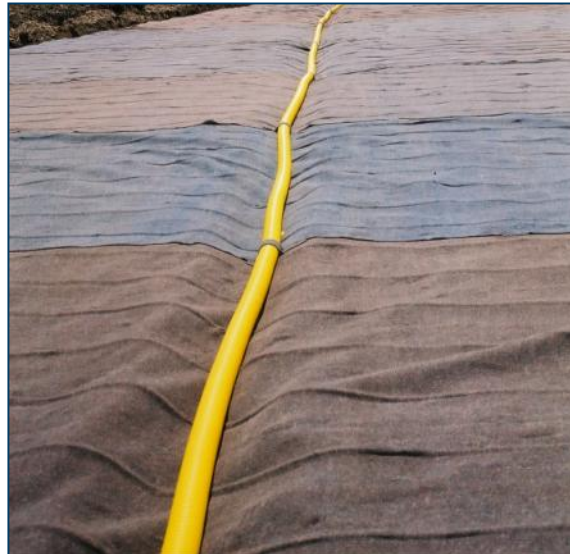
Figure 12: Connection to an interceptor drain
