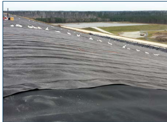
Figure 4: DRAINTUBE™ installation
