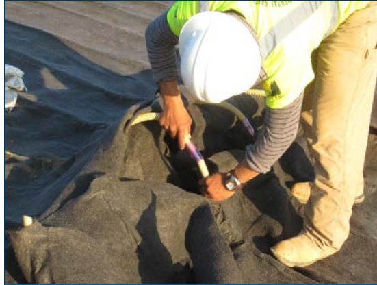
Figure 7: Mini-pipe junction with couplers
