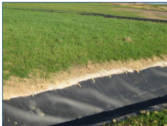
Figure 10: Termination in a ditch
