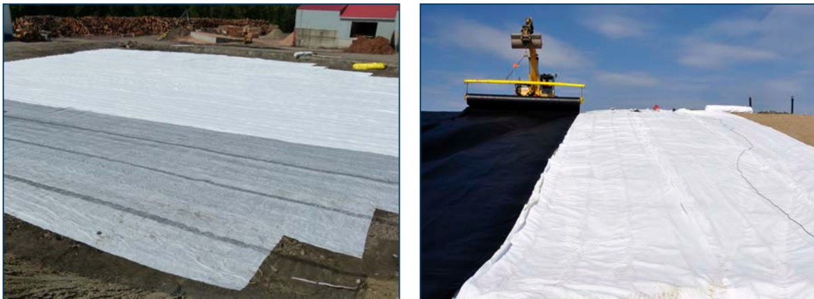
Figures 16: Upper geosynthetic layer placement
