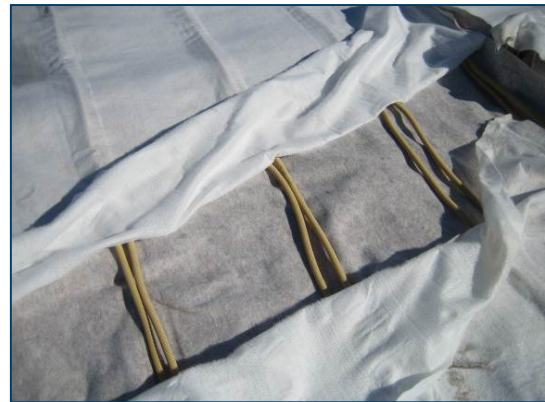
Figures 5: Transverse connections without couplers
