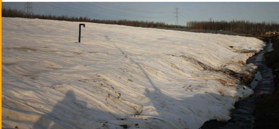
DRAINTUBE™ during installation
