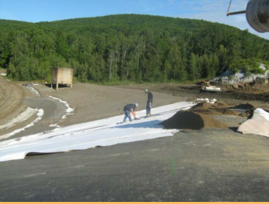
Installation of DRAINTUBE™ - phase 1 - 2008
