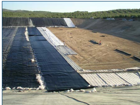
Figures 15: Geomembrane installation
