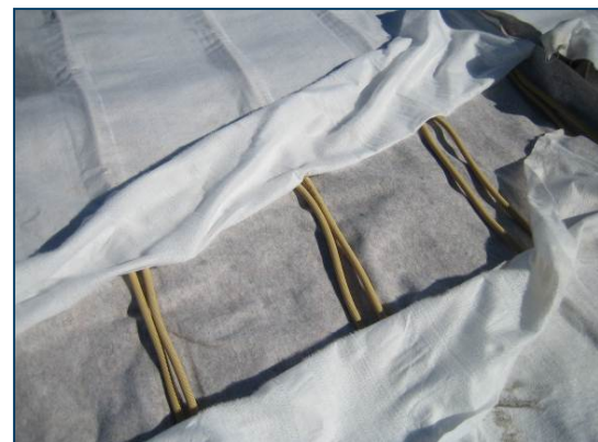
Figures 5: Transverse connections without couplers
