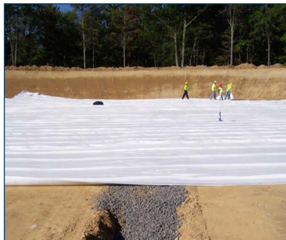
Figures 9: Connection to liquid interceptor drain
