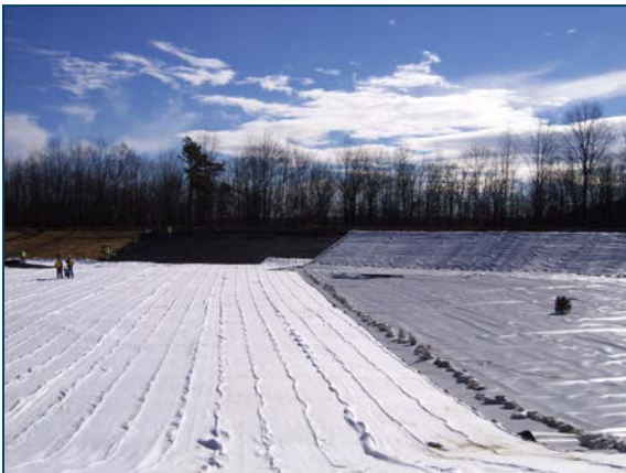
Figures 15: Geomembrane installation
