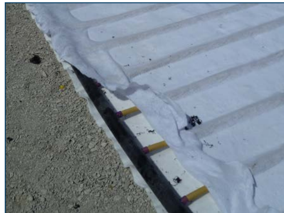
Figures 13: Connection to a plain drain with Quick Connect™
