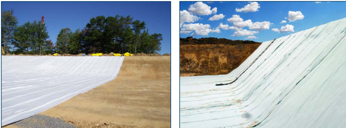
Figure 3: DRAINTUBE™ installation
