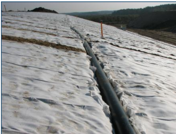
Figures 13: Connection to a plain drain with Quick Connect™
