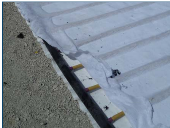
Figures 14: Connection to a plain drain with Quick Connect™
