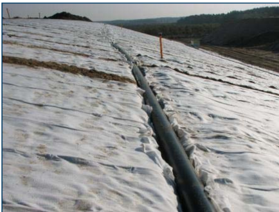
Figures 14: Connection to a plain drain with Quick Connect™
