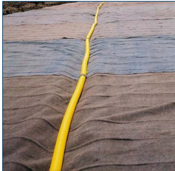
Figure 12: Connection to an interceptor drain
