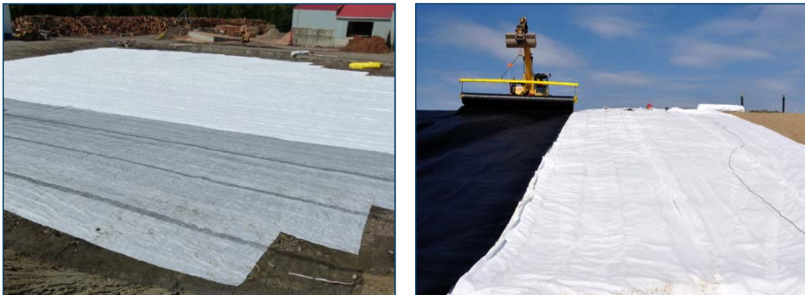
Figures 16: Upper geosynthetic layer placement
