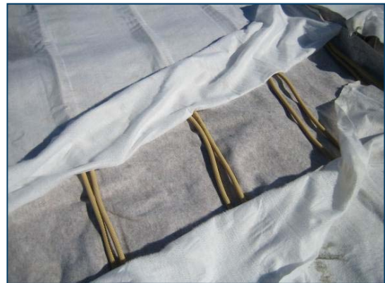
Figures 5: Transverse connections without couplers
