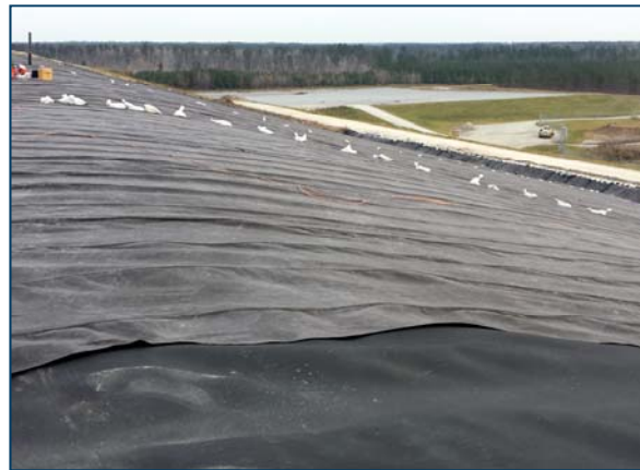
Figure 4: DRAINTUBE™ installation
