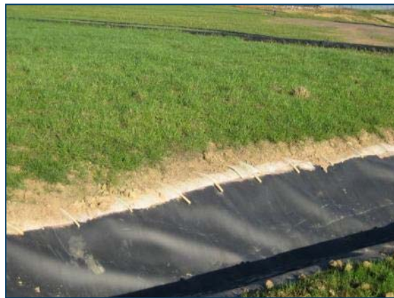
Figure 10: Termination in a ditch
