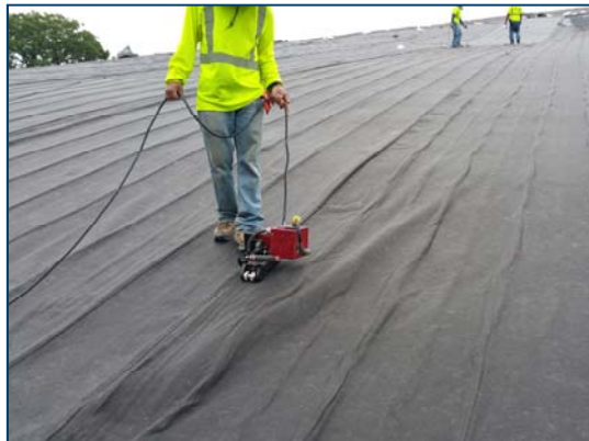
Figure 8: Side by side connections
