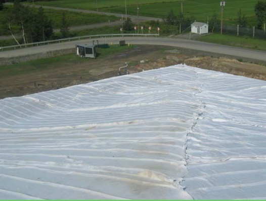
Installation of DRAINTUBE™
