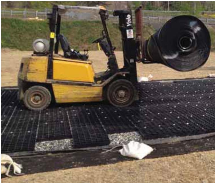
**FIGURE 5** A well pad system that consists of, from the bottom up: a 1.5mm (60mil) HDPE textured geomembrane, a 340 g/m<sup>2</sup> (10 oz./yd<sup>2</sup>) cushion geotextile, a 50mm (2in.) recycled foam product, and a durable, reusable specialty mat product.
