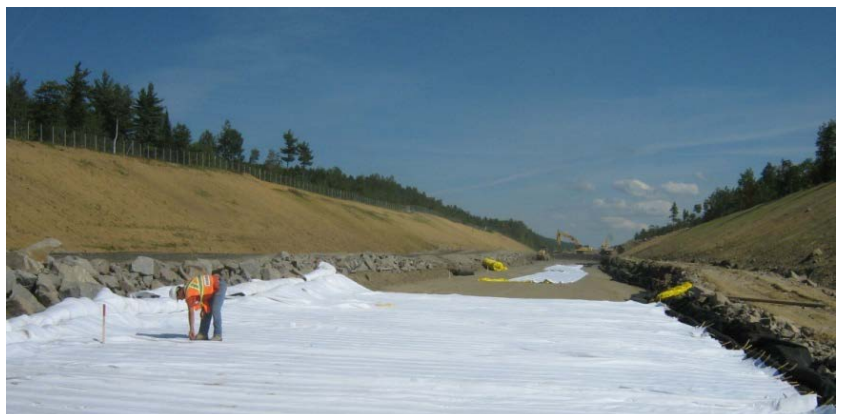
Installation of DRAINTUBE™ on the subgrade – Highway 50
